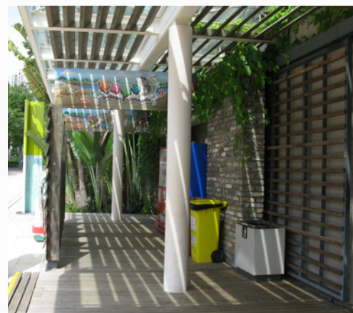
▲ Deep overhang on the roof to shield sunlight
