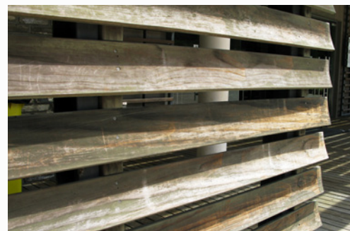
▲ Wooden vertical screens with horizontal louvres installed at the perimeter of the Visitor Centre to screen out sunlight so as to reduce solar heat gain
