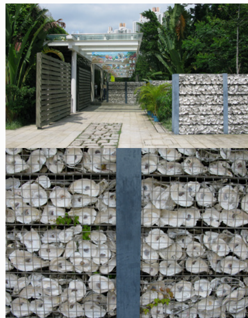
▲ Oyster shell infill wall
