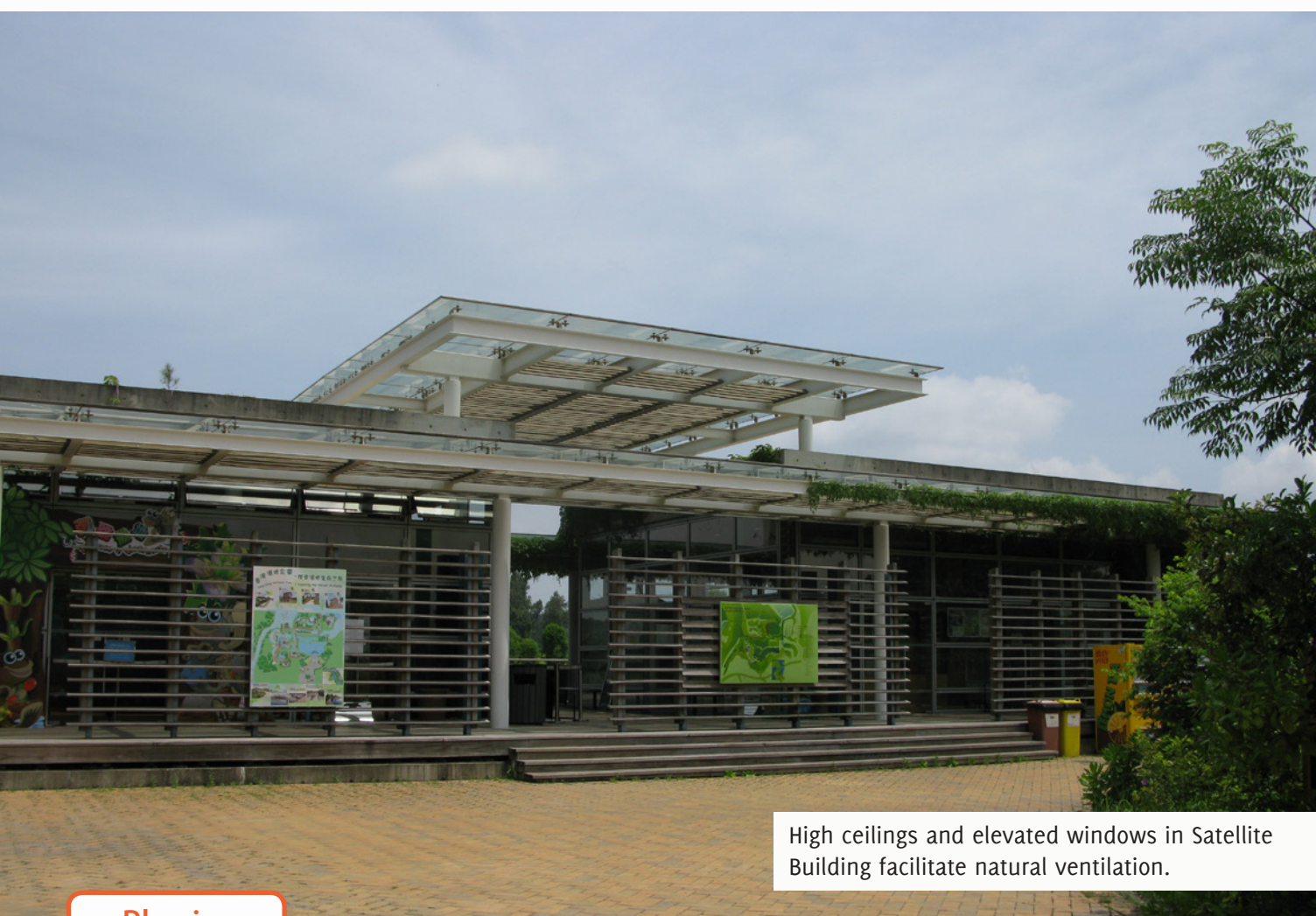
▲ Wooden vertical screens with horizontal louvres installed at the perimeter of the Visitor Centre to screen out sunlight so as to reduce solar heat gain
